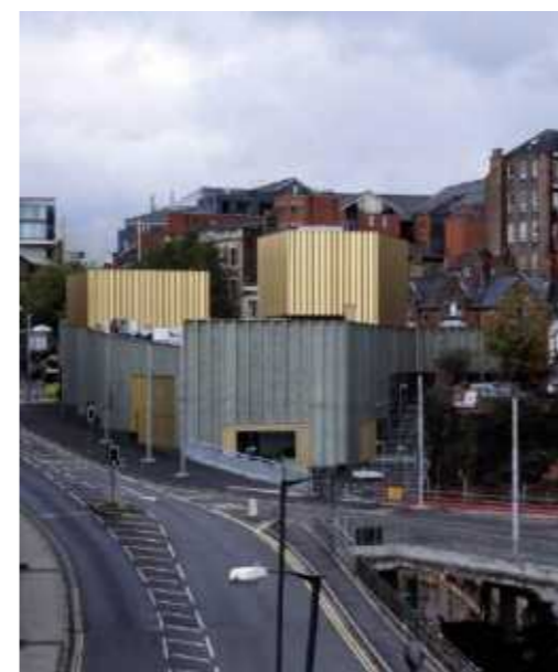
Gallery exterior, the building sits nestled into a steep slope
