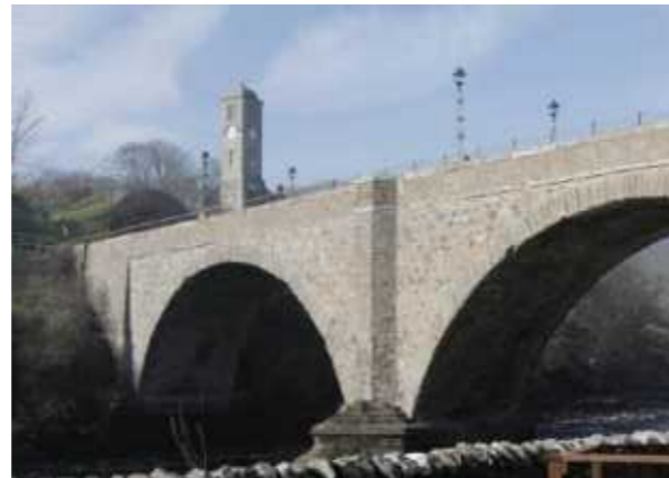
Helmsdale Bridge in coursed rubble
