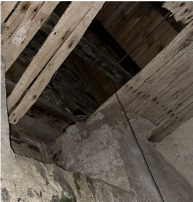
North gable within the Parish Hall attic space
