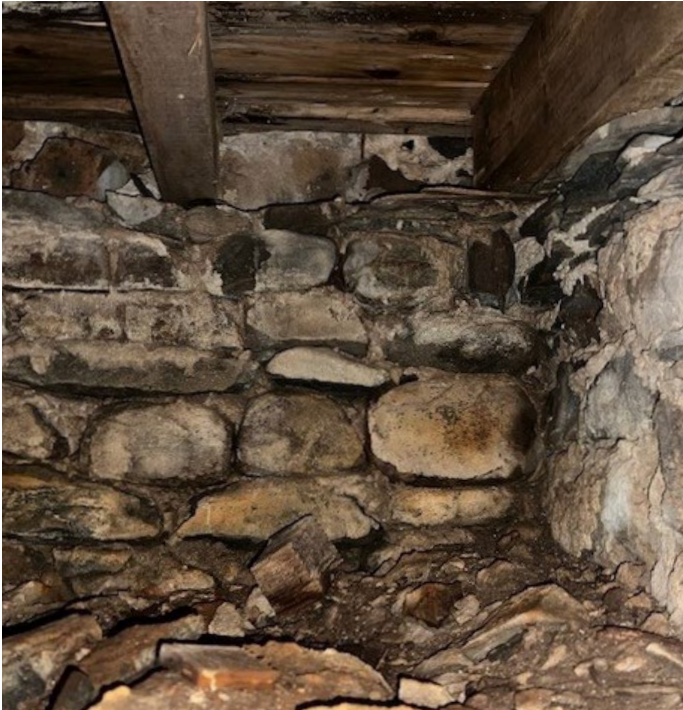
Subfloor below the Vestry
