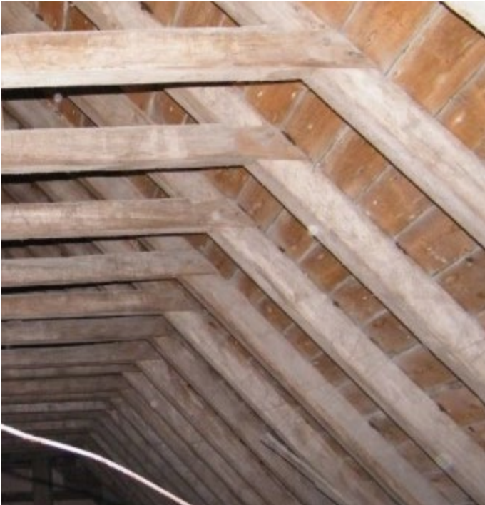
View East in the attic above the Nave
