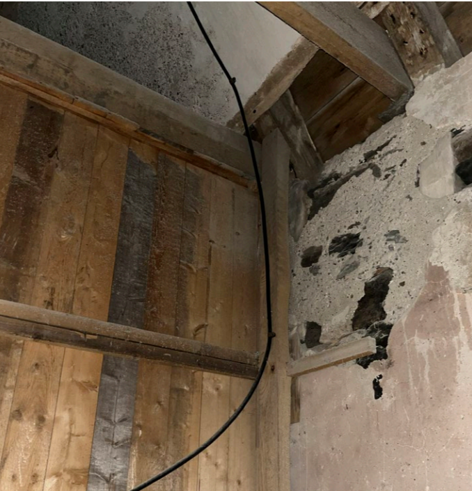
Attic space over the corridor looking South
