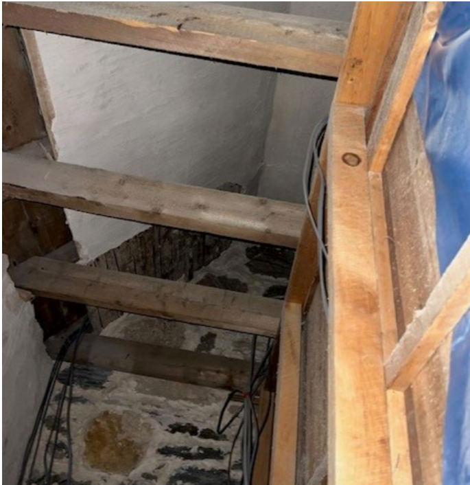
Attic space over the corridor looking North
