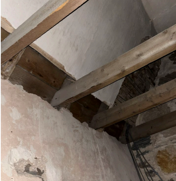
Attic space over the corridor looking North
