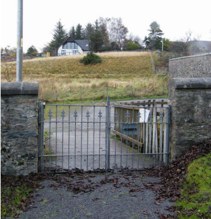
Double gates to the car park
