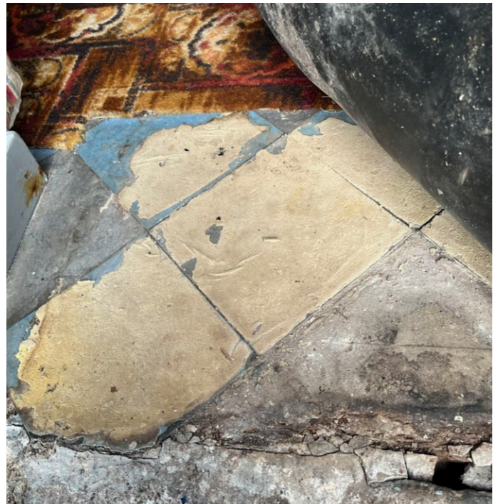
Parish Hall floor
