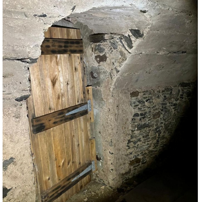
Entrance door as viewed from the burial vault
