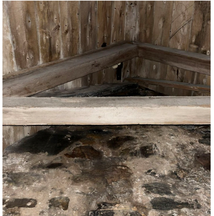
View West towards the West gable
