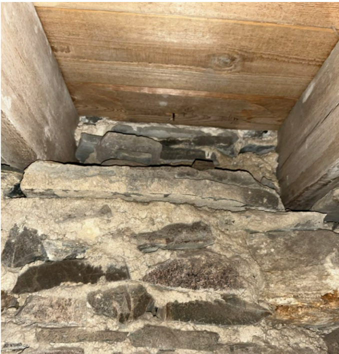
Solum, floorboards and joists appear dry
