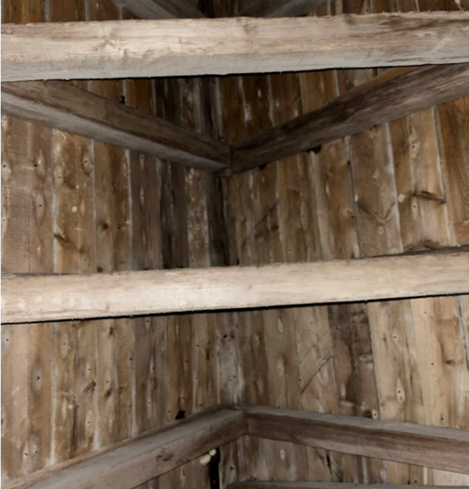
View up to the ridge in the attic above the Nave
