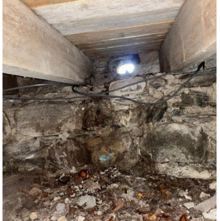
Open solum vent in the external wall (04.09.2025)
