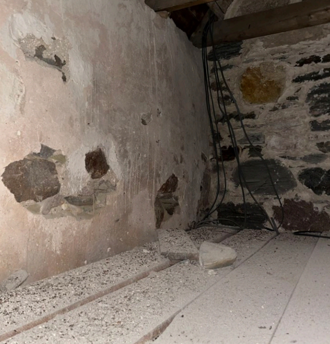
Attic space over the corridor looking North
